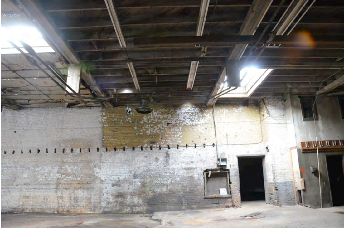
Photo 11 – Looking West Toward West Wall and Door to 1980 Addition
