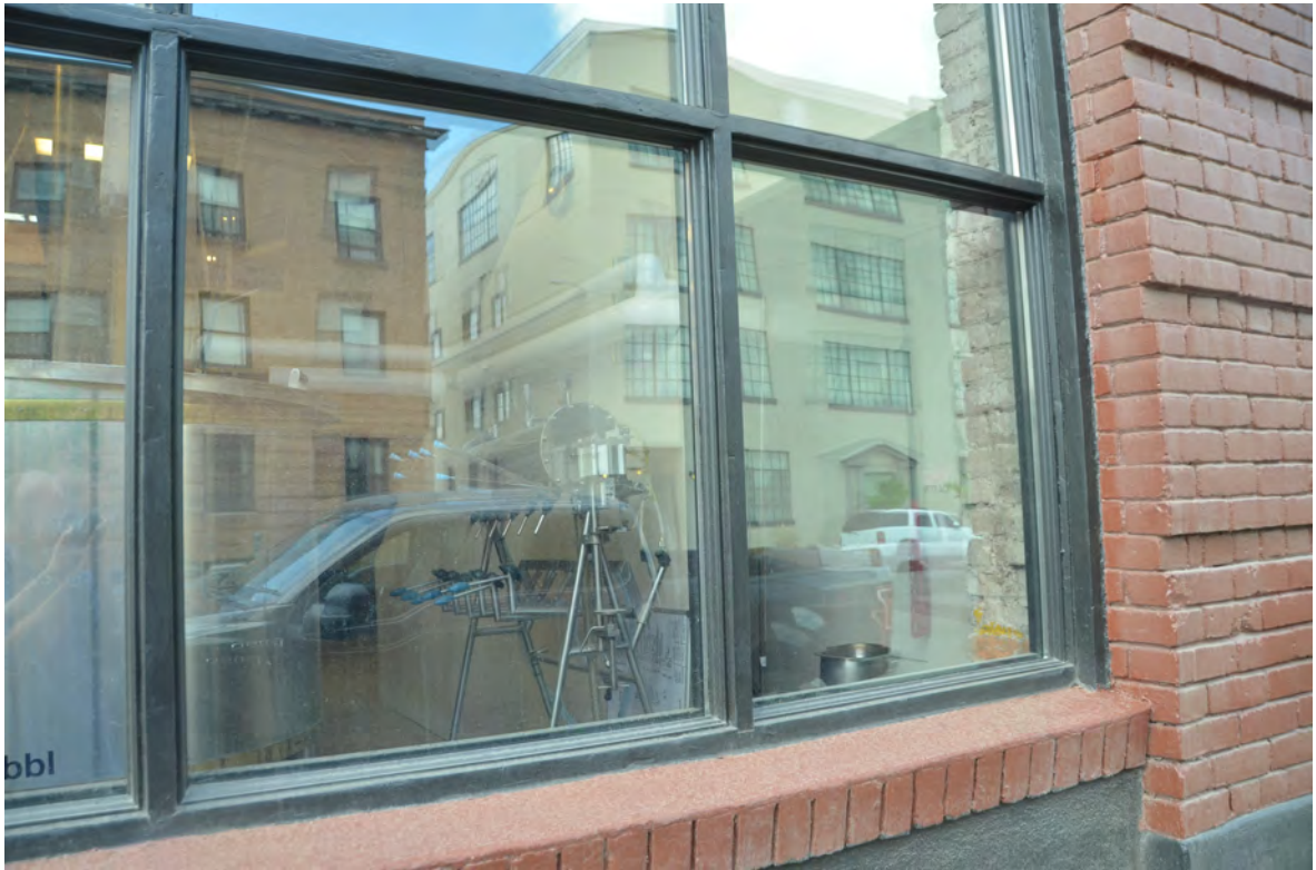
Photo 13 – East Façade –Detail of Refurbished Original Wood Sash and Brick Sill
