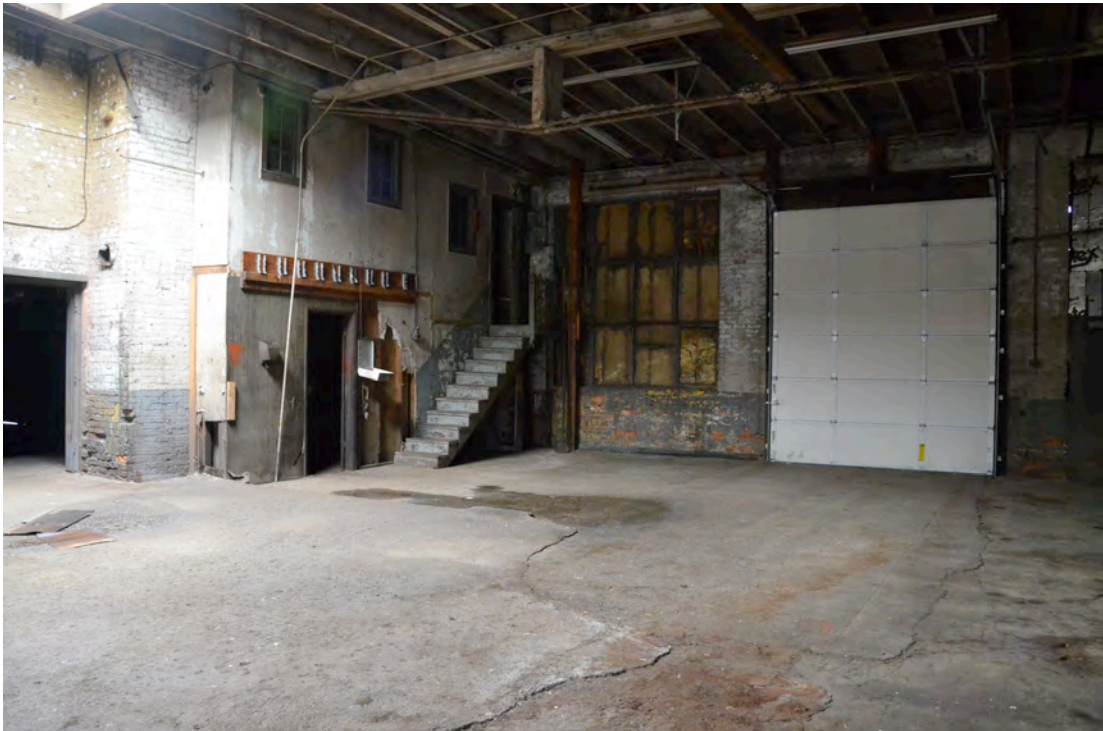
Photo 10 – Looking NW at NW Corner of Garage & Former Mezzanine
