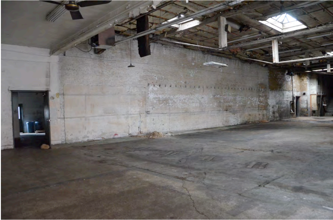
Photo 9 – Looking Northwest at West Wall with Door Opening to 1980 Addition
