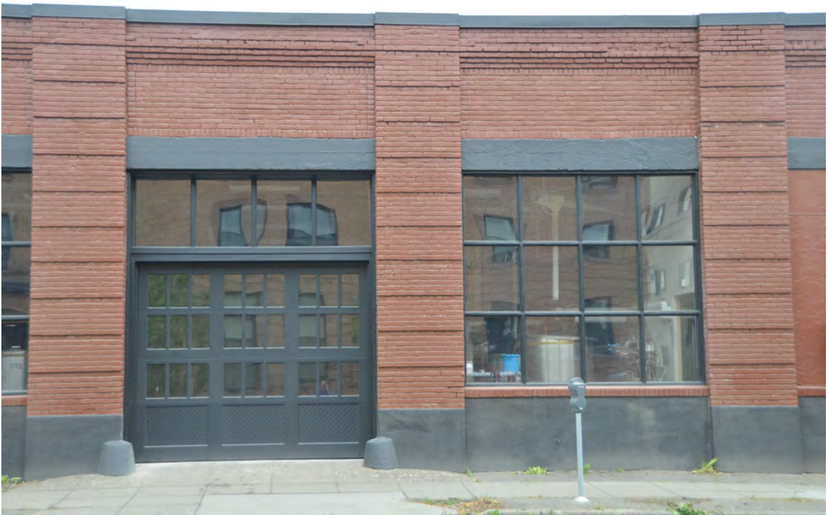
Photo 10 - East Façade, Showing Bays 7 and 8
