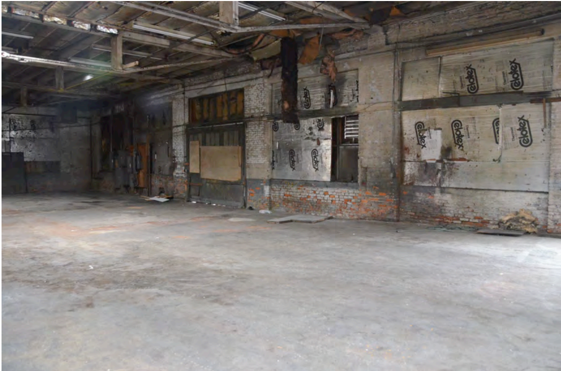
Photo 14 – Looking NE Toward NE Corner Showing Bays 7, 6 & 5
