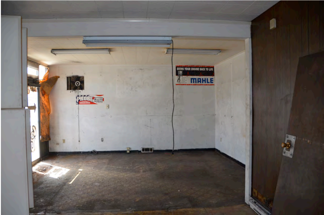
Photo 3 – Looking West Across Front Office to Front Entry
