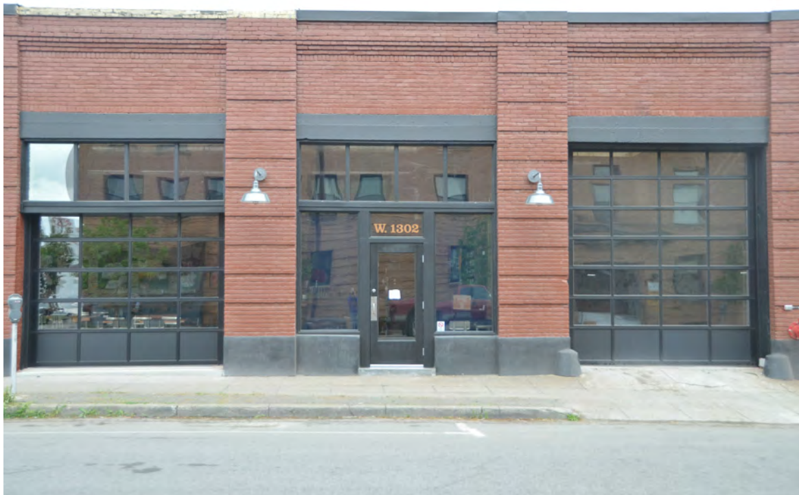
Photo 8 - East Façade, Showing Bays 2, 3 and 4
