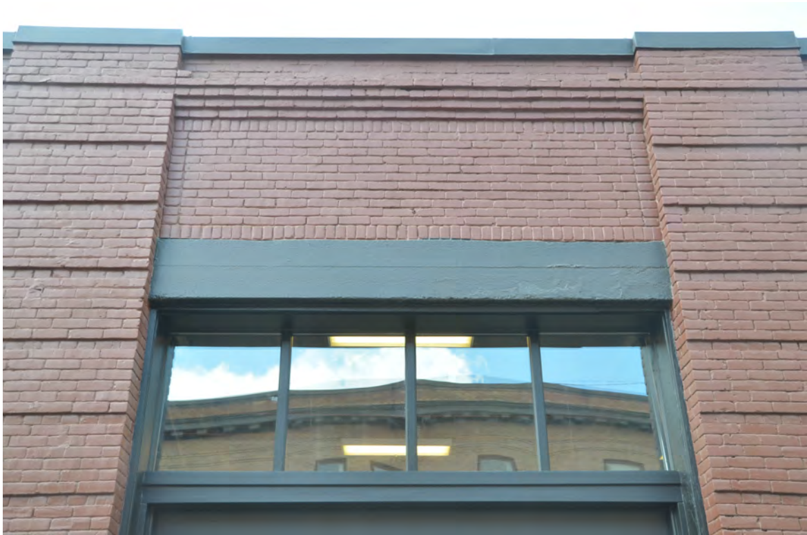
Photo 12 – East Façade Showing Refurbished Original Transom Sash & Parapet
