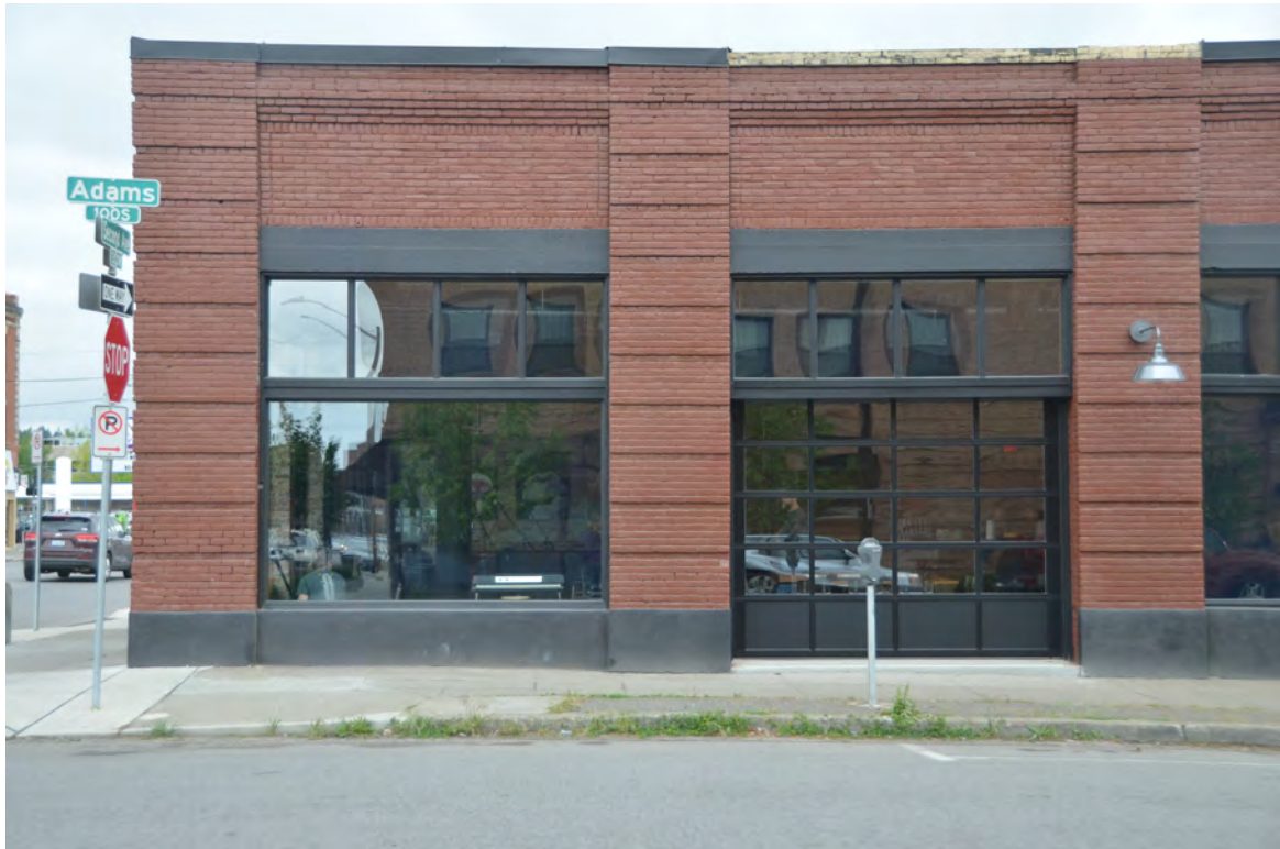
Photo 7 – Looking West Showing East Façade Bays 1 and 2
