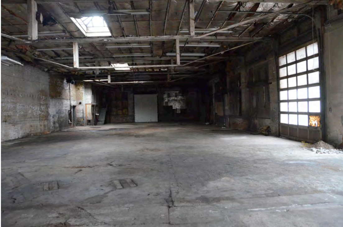
Photo 7 – Looking North Across Garage (Toward Rear and Alley)
