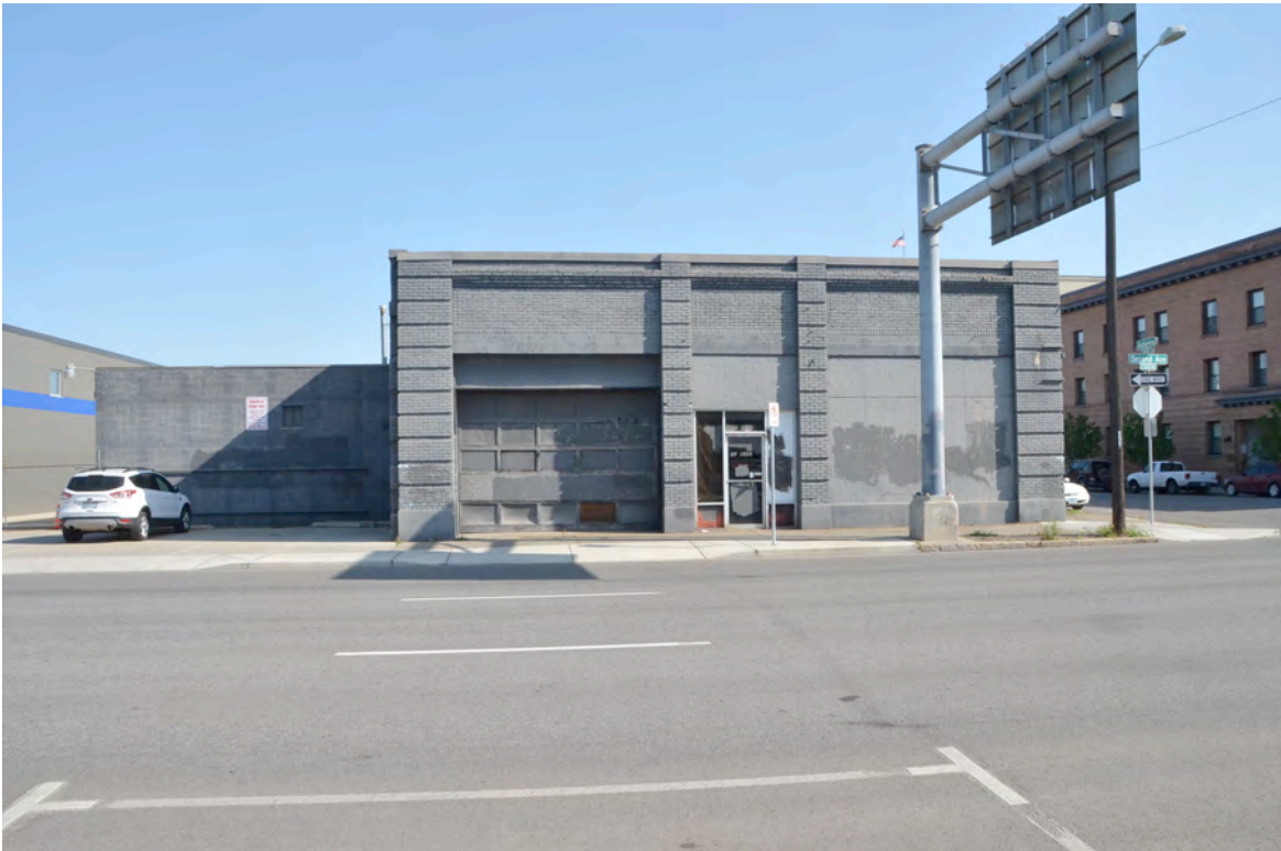
Photo 1 – View to North Showing Front Façade of 1302 West 2 nd Avenue (Building Built ca. 1921; Addition 1980)
