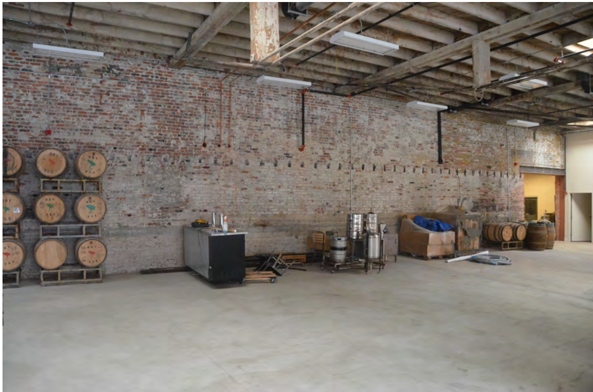
Photo 8 – Looking West Toward West Wall and Door to 1980 Addition (Brewery)
