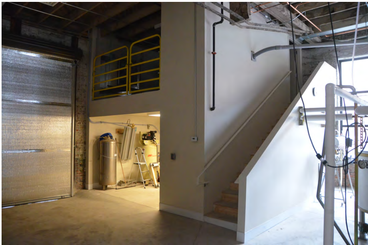
Photo 10 – Looking Toward NE Corner, New Mezzanine and Equipment Room and Rear Shop Door
