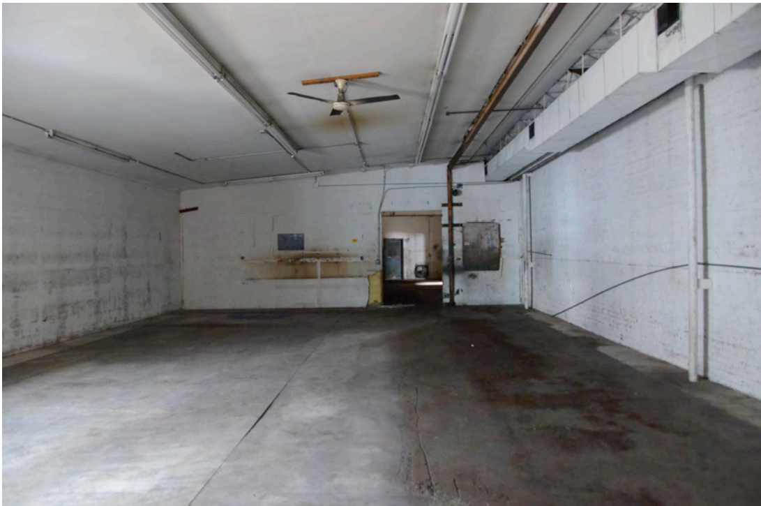
Photo 18 - Looking North Across 1980 Addition (Southerly Room)
