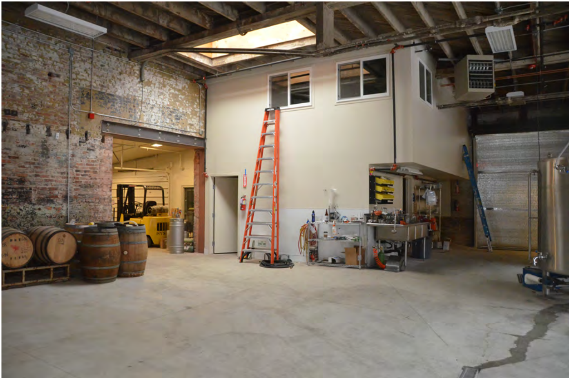
Photo 9 – Looking Toward NW Corner, New Mezzanine and Rear Shop Door
