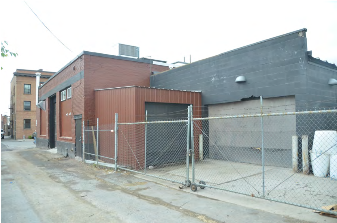
Photo 6 - View to SE Showing Rear Façade (northwest corner) and West Side Addition
