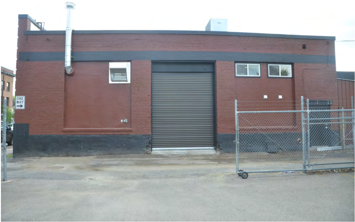
Photo 5 – Looking South at Rear (North Façade)
