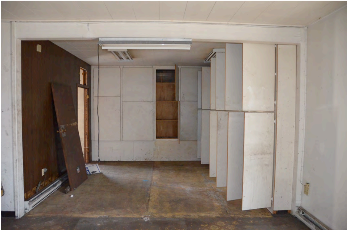
Photo 2 – Looking East Across Front Office Toward SE Corner (Bay 1 Covered Over)
