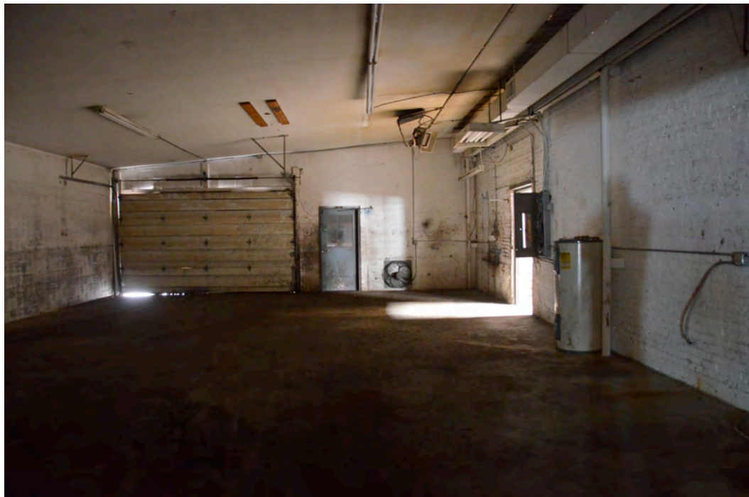
Photo 20 - Looking North Across 1980 Addition (Northerly Room)
