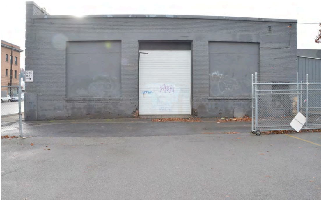
Photo 5 – Looking South at Rear (North Façade)
