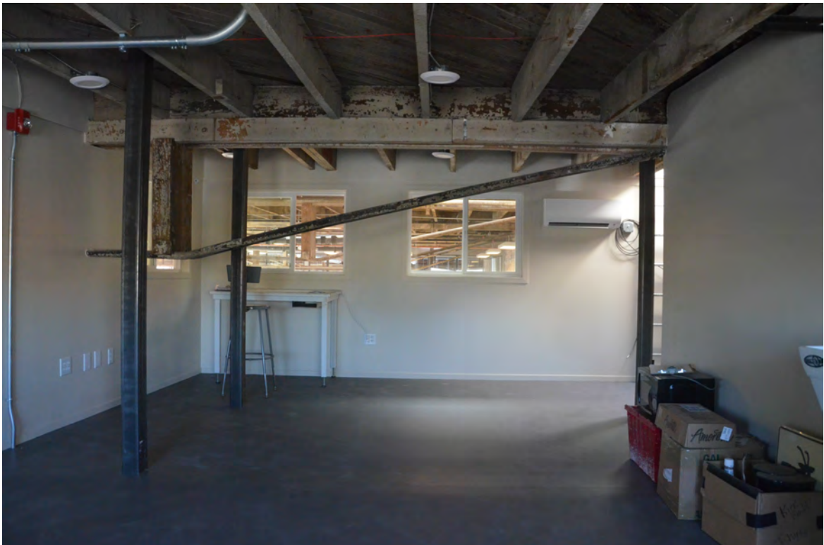
Photo 20 – Office in Mezzanine with Access Ladder to Roof
