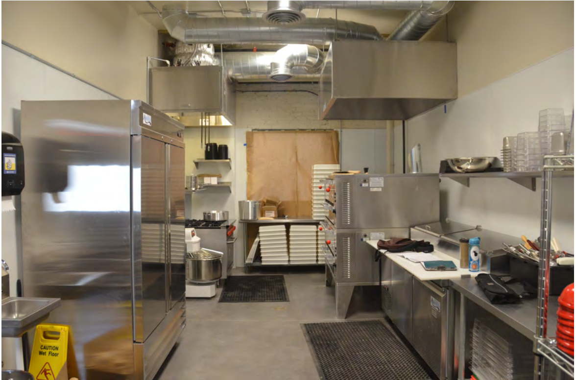
Photo 15 – New Kitchen in 1980 Addition
