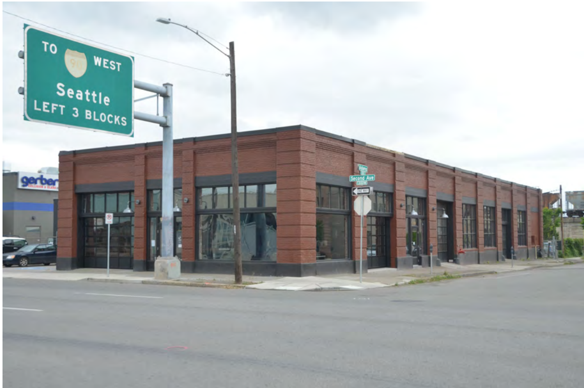
Photo 3 – View to Northwest Showing Front /Façade and East Facade
