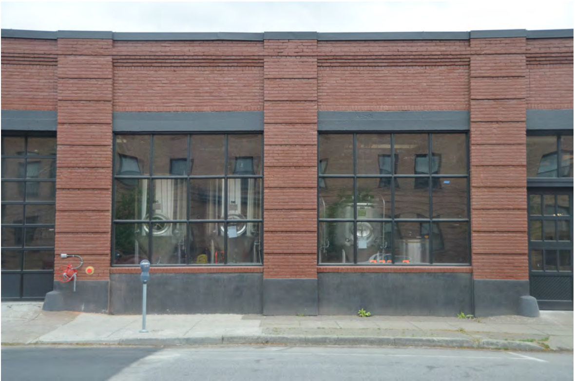
Photo 9 - East Façade, Showing Bays 5 and 6
