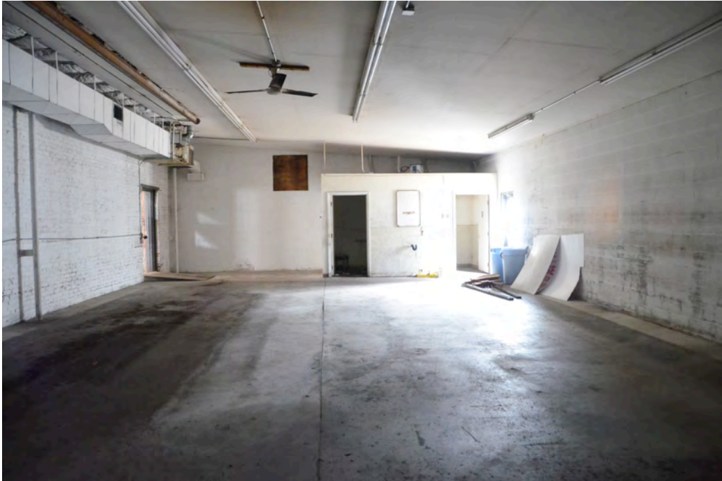
Photo 19 - Looking South Across 1980 Addition (Southerly Room)
