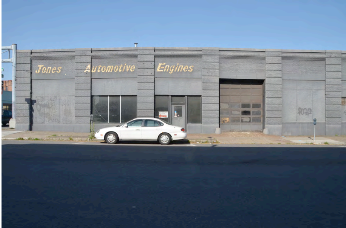
Photo 7 – Looking West Showing East Façade Bays 1 through 5
