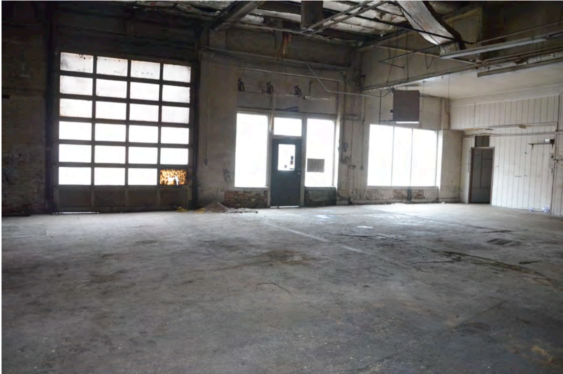
Photo 15 – Looking SE Toward Bays 4, 3 & 2 and Office in SE Corner
