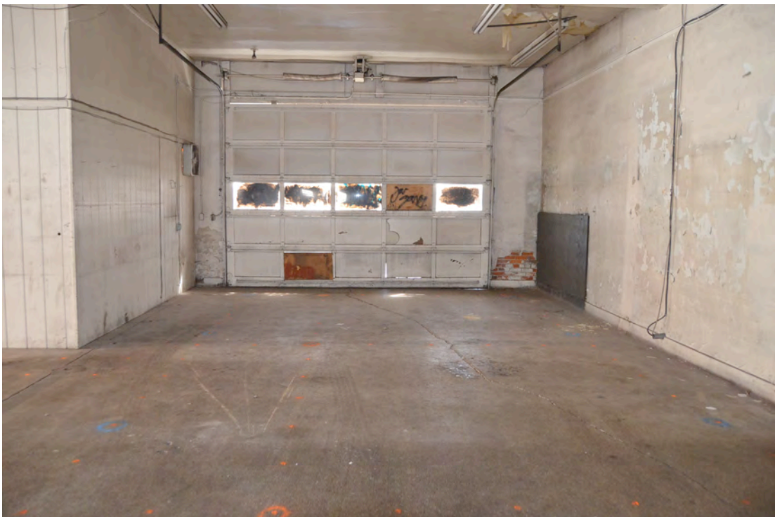
Photo 6 – Looking South Showing Front Garage Door (SW Corner)
