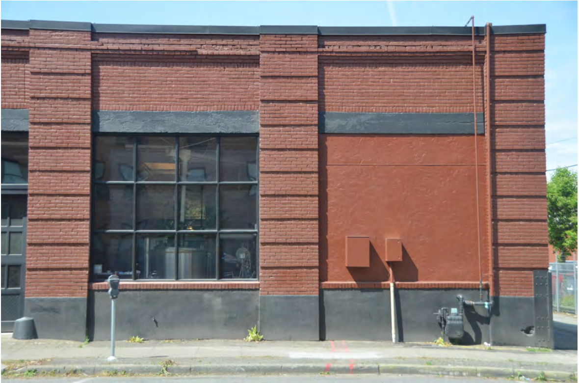
Photo 11 - East Façade, Showing Bays 8 and 9
