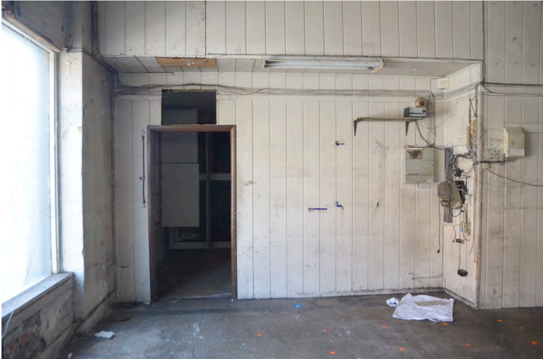
Photo 5 – Looking South Toward Door to Office (SE Corner)
