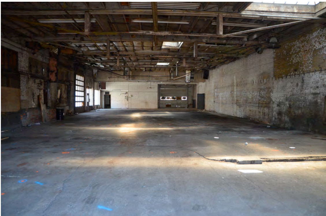
Photo 8 – Looking South Across Garage (Toward Front and 2 nd Avenue)
