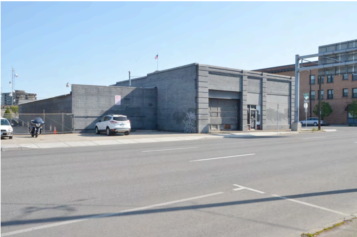
Photo 2 – View to Northeast Showing Southwest Corner and Addition
