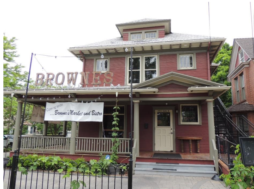
The house at 1928 W Pacific Avenue has experienced adaptive re-use, changing to commercial uses over time.
