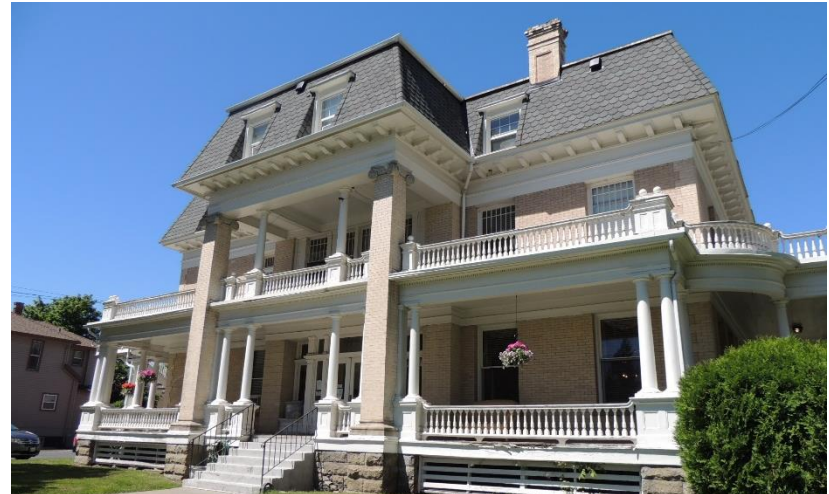
2308 W 3rd Avenue contributes to the Browne's Addition Historic District.
