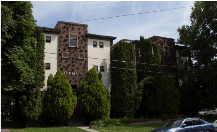
Osmun Apartments (1814-1818 W 1 st Avenue), displaying buildings that are close together with only facades that are highly visible.
