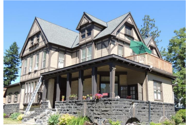
2108 W Pacific Avenue retains its original mix of half-timbering and wood lapped sidings.
