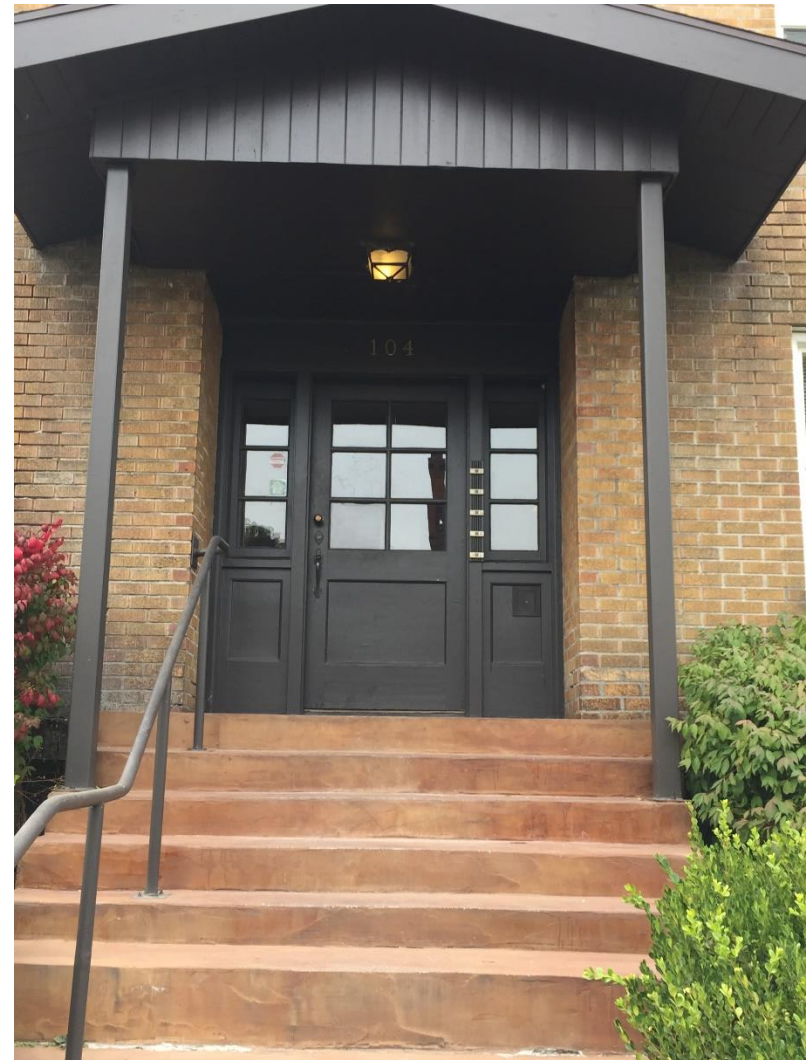
104 S Oak Street (above) and 1824 W Riverside Avenue (at left).
