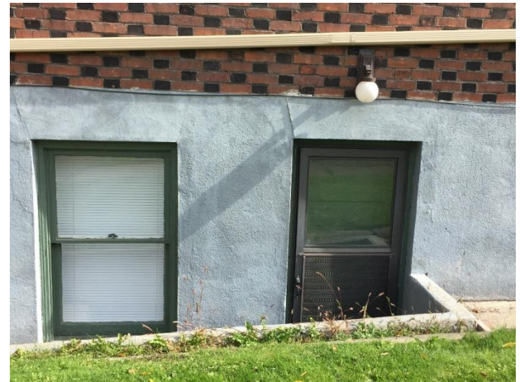
Parged basement level with outline of lintels above openings visible.
