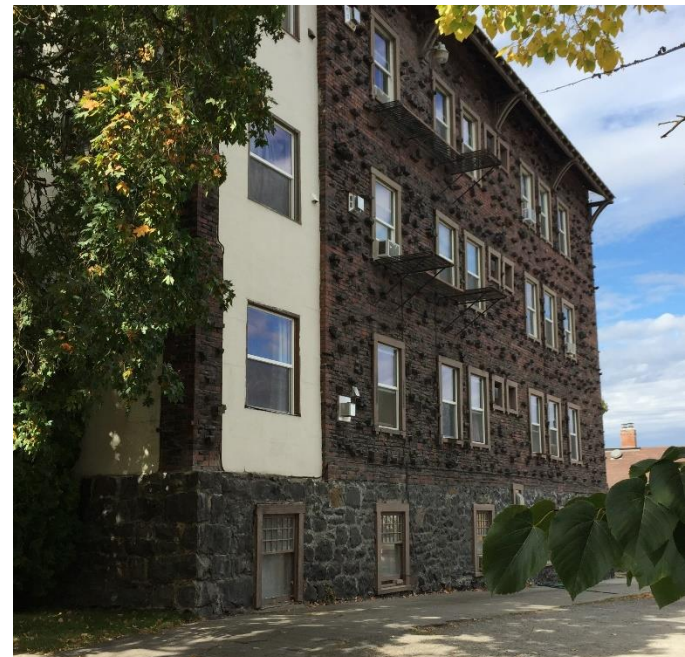
East side of Osmun Annex is highly visible because of parking area.
