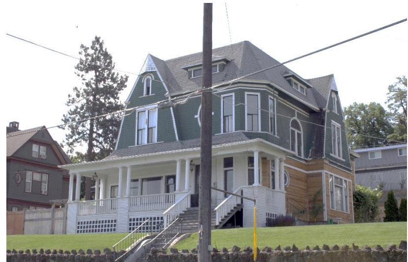
The siding on 2027 W Riverside Avenue has been restored to period-appropriate materials and design.
