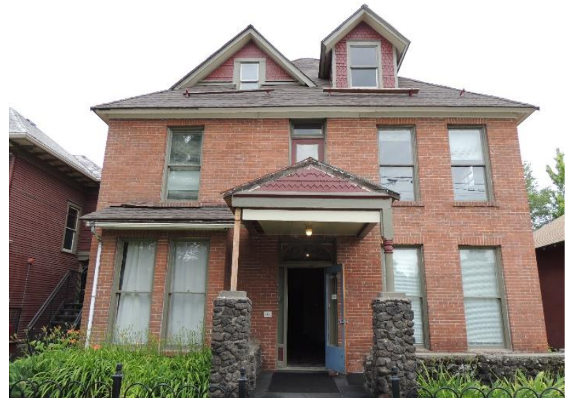
The porch on 1924 W Pacific Avenue has been modified over time.
