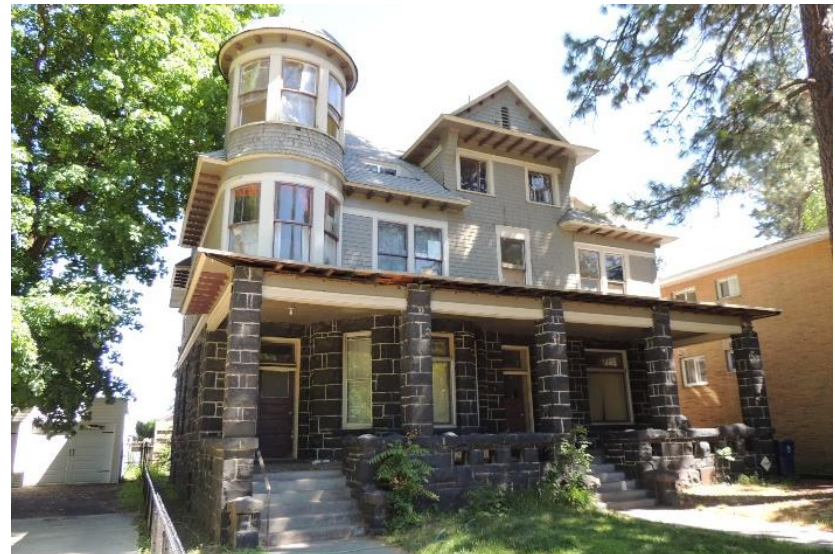
Both 23230 W Pacific Avenue (above) and 2208 W Pacific Avenue (below) exhibit original masonry porch posts and railings.
