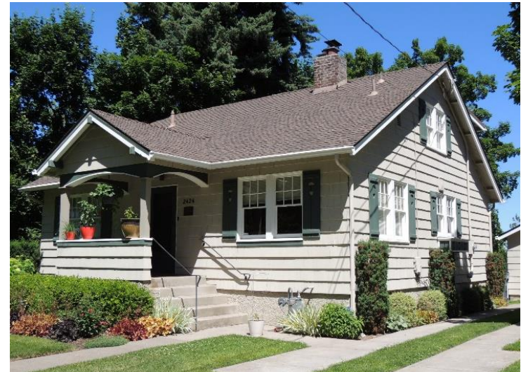
2424 W Pacific Avenue rests on a raised poured concrete basement.
