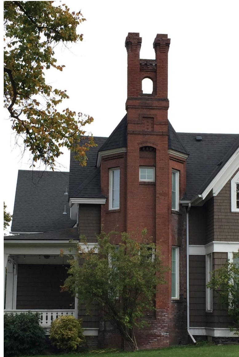
1725 W 1st Avenue has the most distinct corbeled brick chimney in Browne's Addition Historic District.
