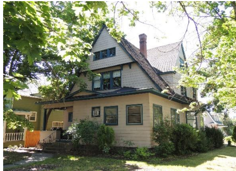
Most of the front porch on 1927 W 2nd Avenue has been enclosed.
