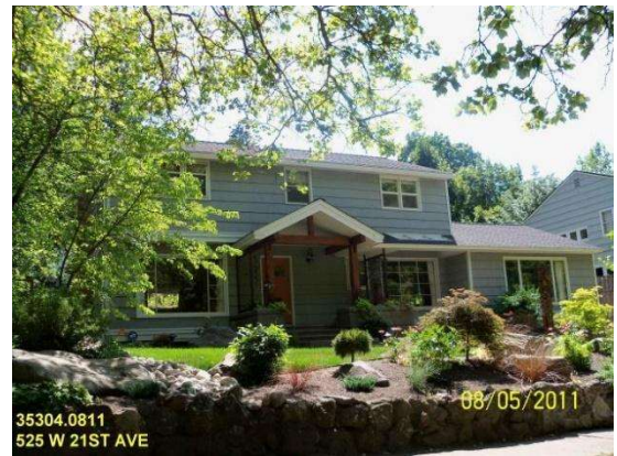
525 W 21 st Avenue 1950 35304.2111 628 W 19TH AVE
