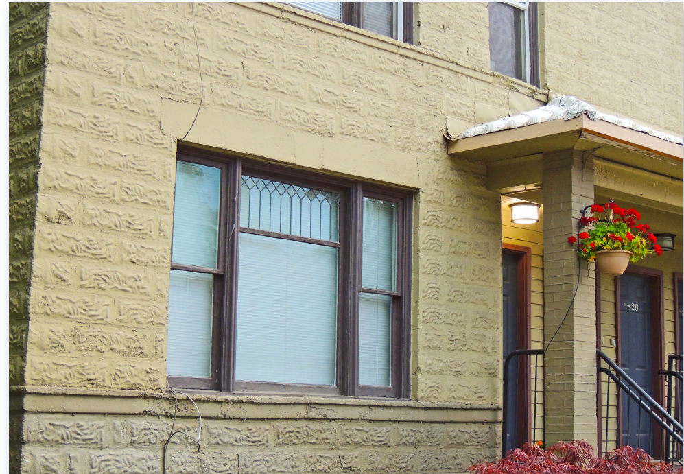
Windows at the small apartment building at 820 S Monroe are intact and include a decorative leaded glass transom.
