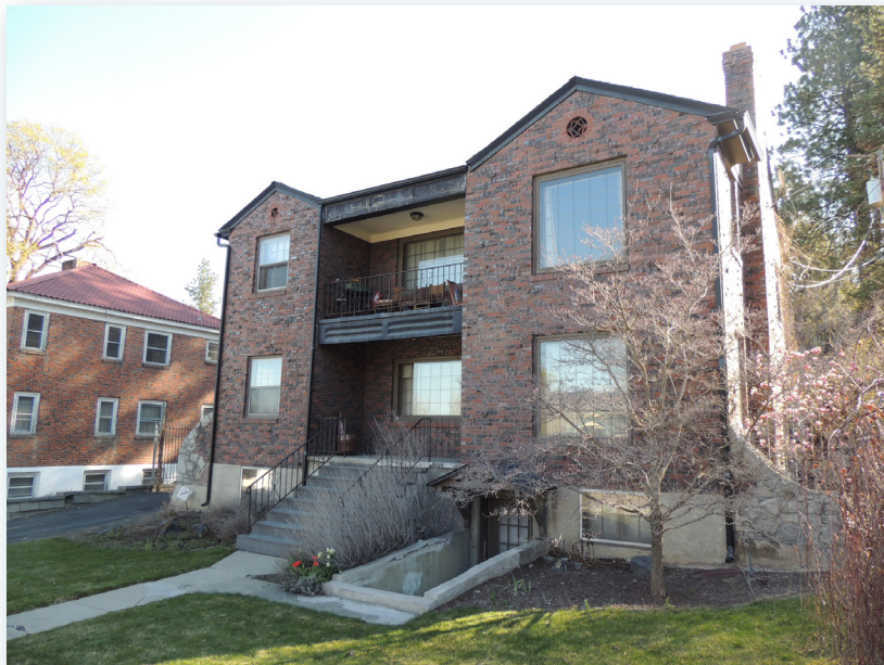
The small apartment building at 1023 S Monroe retains very good integrity except for the replacement of windows on the main facade. Right: The building in 1940, photo courtesy of the NWMAC L87-1.19183-40.
