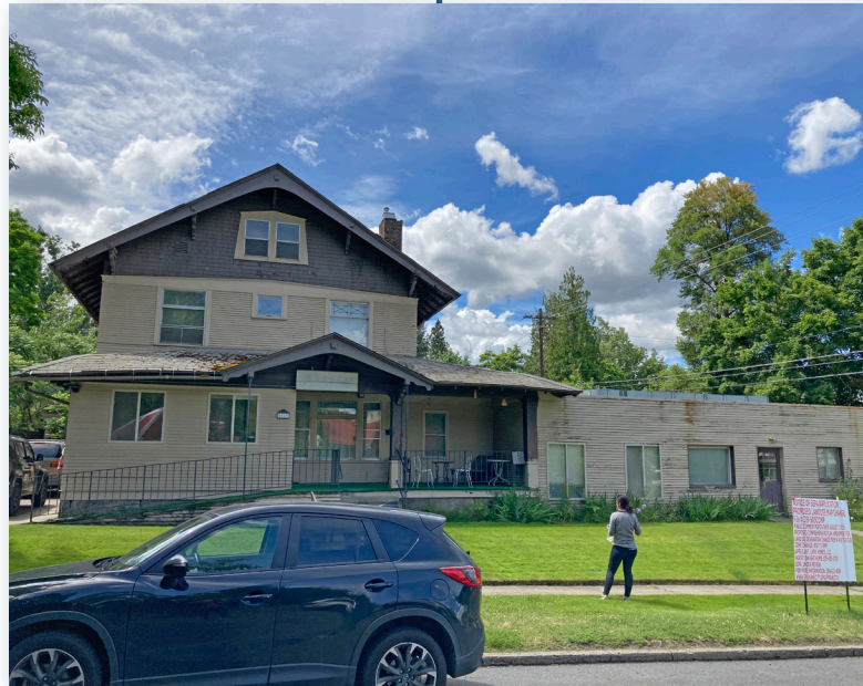
This house at 1117 W Tenth Avenue had a large, incompatible addition added in the 1950s when it functioned as a nursing facility.
