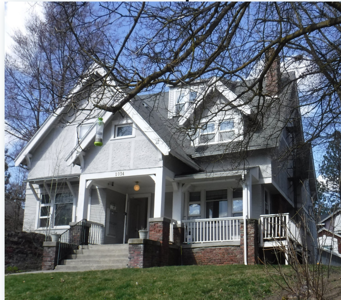
1034 W Eighth Ave: This house has a steeply pitched cross gable roof.
