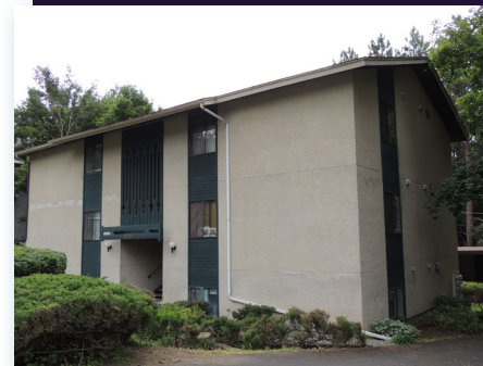
Vertical Plane Breaks at 909 W Thirteenth
