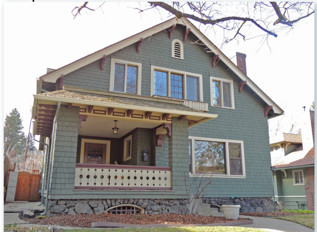
919 W Twelfth: Partial width front porch with nearly solid decorative balustrade, shingled columns and deep eaves accentuate this attractive home.
