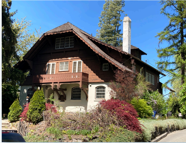
This home at 1034 W 7th Avenue has many architectural features including arched lintels, multiple mullion and muntins on the windows and a clipped gable roof.
