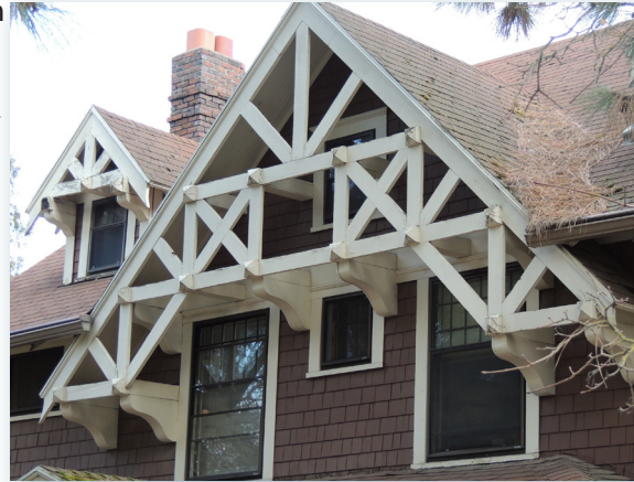
The house at 1014 W Twelfth Ave has shingle siding and interesting stick detailing on the gable ends.
